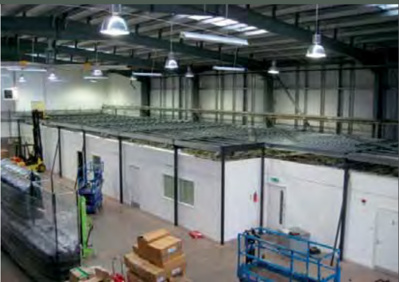
MEZZANINE FLOOR INSTALLATION
